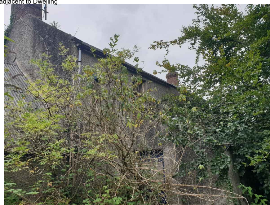
P12: North / East Rear Elevation of Dwelling
