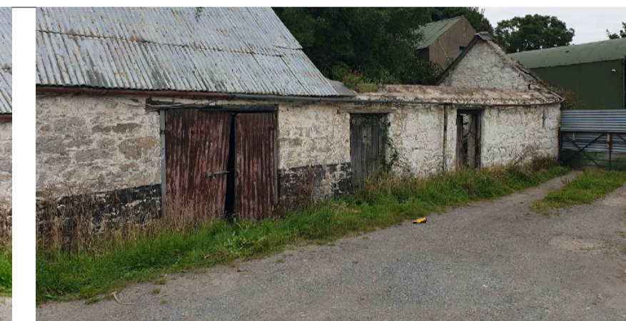
P9: South / East Elevations Third Outhouse in Courtyard
