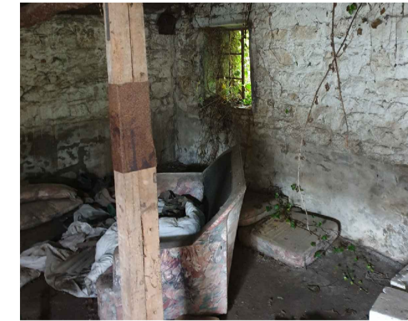
P14: Inside of Third Outhouse with crittall window in background
