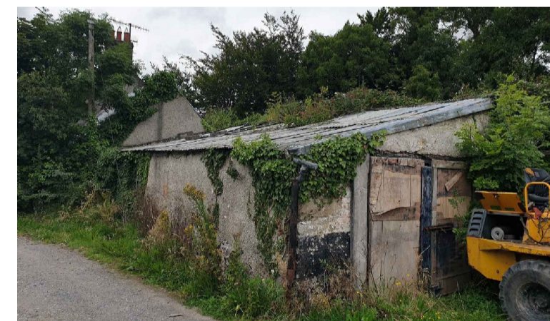
P7: West Elevation Second Outhouse in Courtyard
